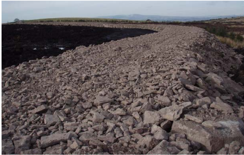
Figure 14.5: Rockfill Peat Repository on an Existing ESB Wind Farm
