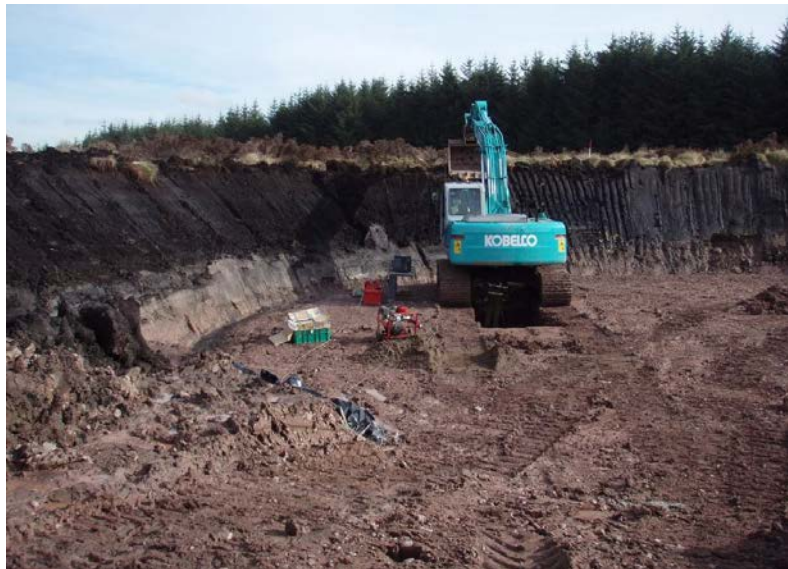
Figure 14.6: Turbine Excavation Trimmed Back to a Stable Temporary Side Slope
